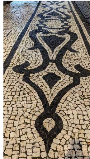
These are all hand cut and laid.
